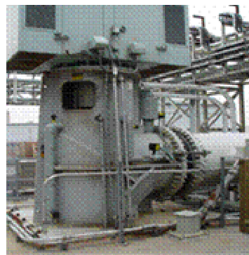
Fig. 11: Motor stand for large vertical pump installation.
