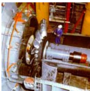
Fig. 12 Large fan installation
